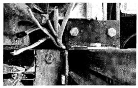
Fig 8. Structural columns and beam also function as conduits for electrical and plumbing systems in the open grid system
