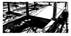
*Fig. 9. Beams and columns serve as a utility grid and to support the floor inserts*
